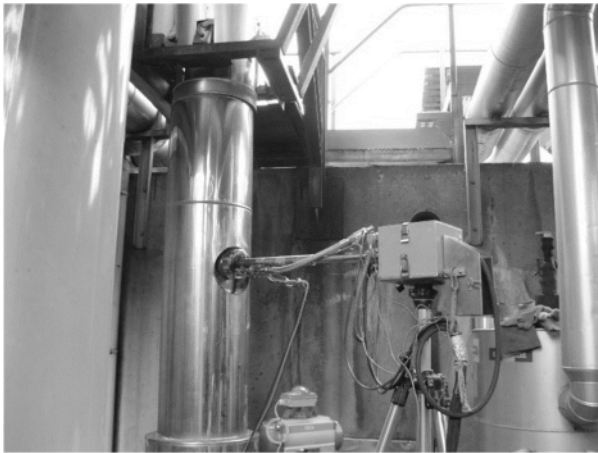
Figure 2. Gas sampling in engine exhaust line
