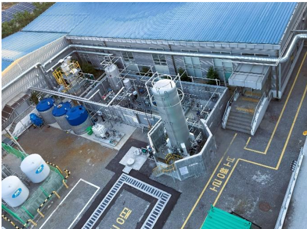
Figure 2. Ammonia fuel storage and supply system of Korean Register's test center
