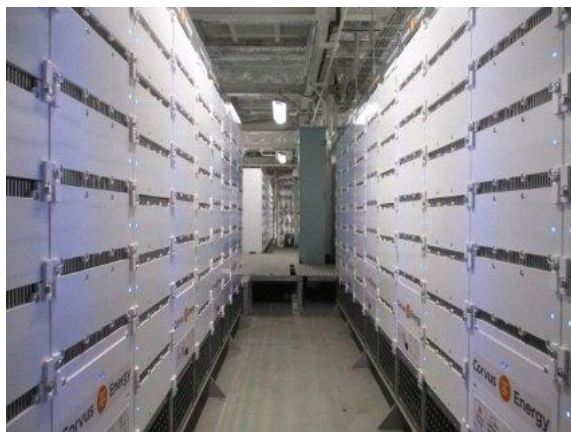
Figure 9. Lithium-ion battery room
