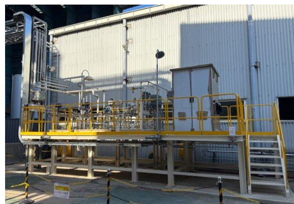
Figure 1. Hydrogen supply skid system.
