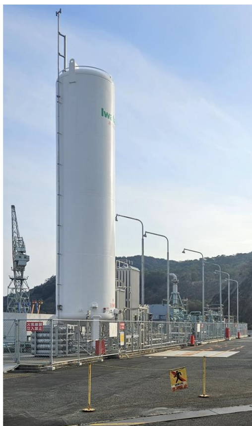
Figure 1. Picture of the hydrogen supply system showing the liquid hydrogen storage tank, vaporisers, and compressors.
