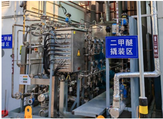
Figure 3 Dimethyl ether supply system
