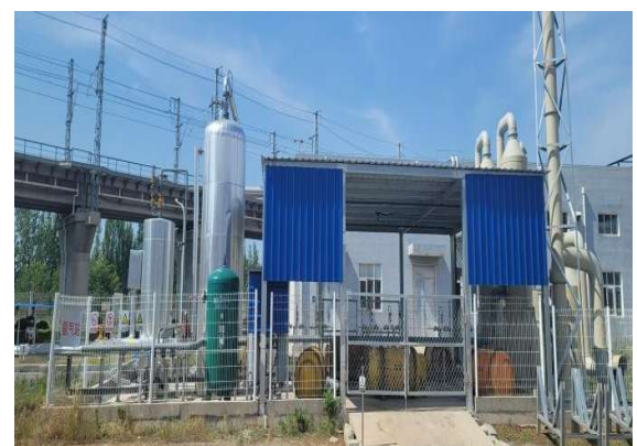
Figure 6. Ammonia Station for supply to test-cell
