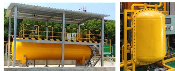
Figure 9 The ammonia supply system of the \text{NH}_3 /diesel dual-fuel SCE
